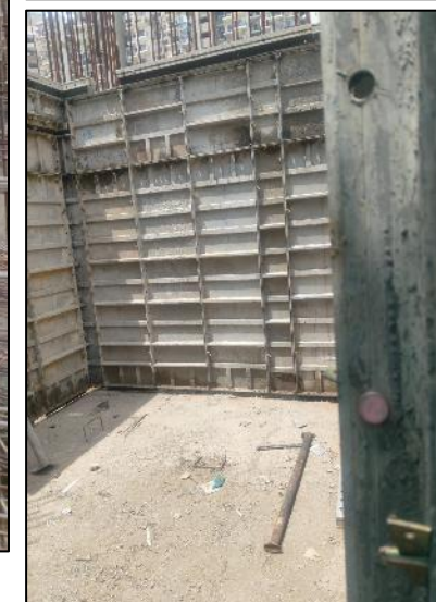
Shuttering work in progress
