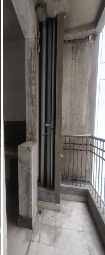
Vertical Stacks-Plumbing Shafts
