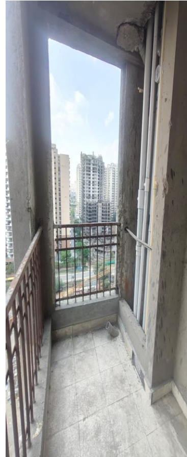
Vertical Stacks-Plumbing Shafts
