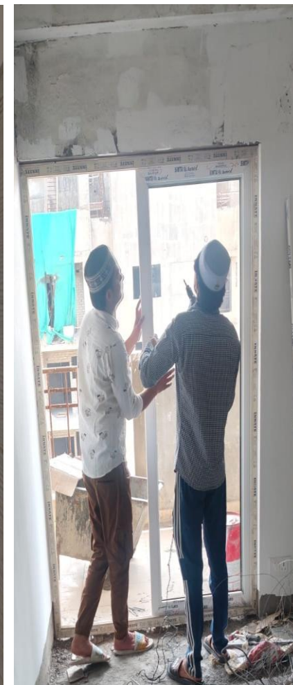
Upvc door fixing in progress
