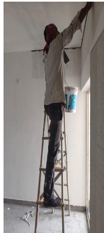
Painting work in progress
