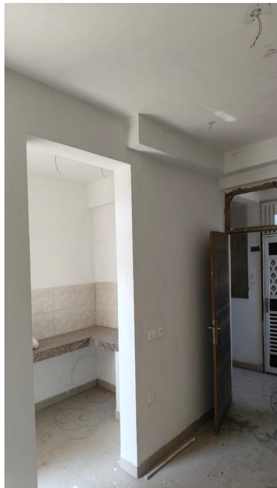
Electrical Switch & Wiring Work in Progress
