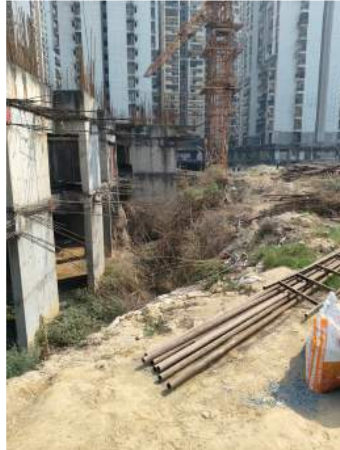
Tower P & Surrounding NTA
