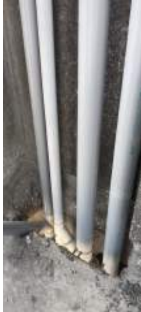
Vertical Stacks-Plumbing Shafts
