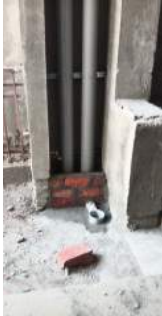
Vertical Stacks-Plumbing Shafts
